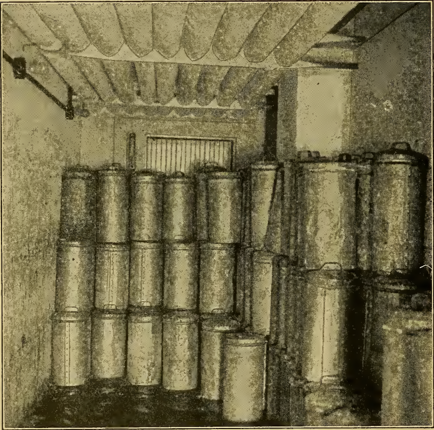
FIG. 56.—Forced-air hardening-room.
